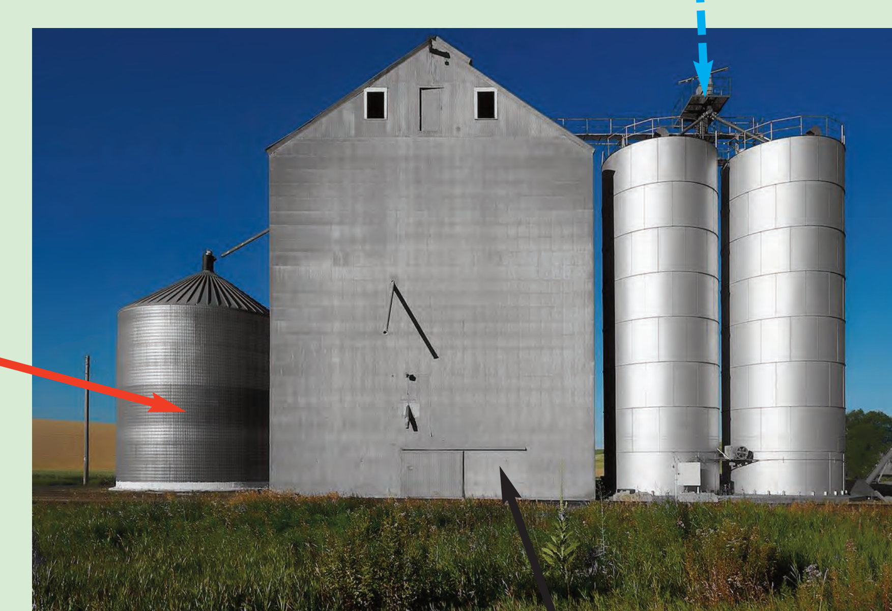
The Server Farm (double redundant)
